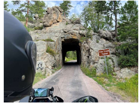
Iron Creek Tunnel
